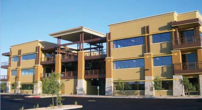
BELL & REEMS PROFESSIONAL OFFICES SURPRISE, ARIZONA
