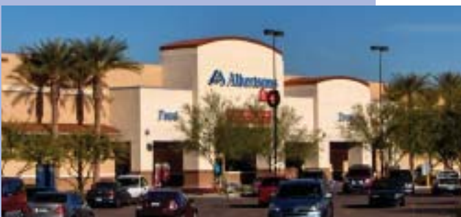
COPPERPOINT CENTER CHANDLER, ARIZONA
