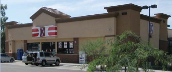
CIRCLE K CONVENIENCE MART TEMPE, ARIZONA
